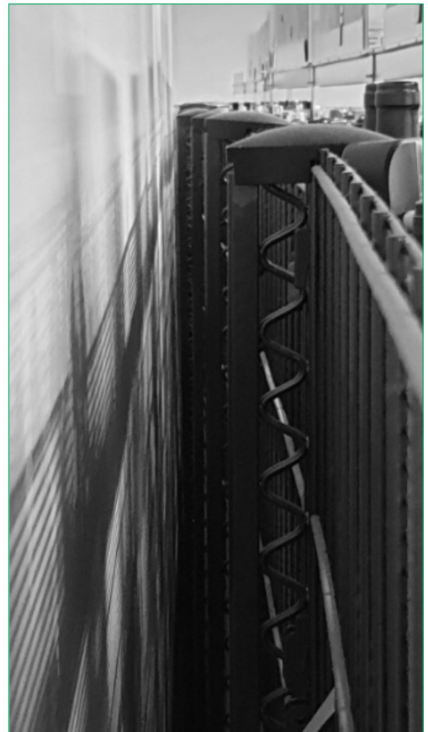
Ignoring installation instructions can have catastrophic effects, This unit is flexing under load.
